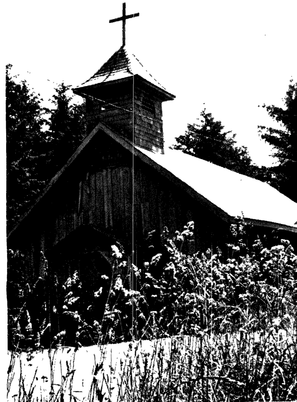
FROM THE PAST--This old Shaker Church built in 1917, served LaPush for more than 45 years, both as a house of worship and a community hall. Standing somewhat unstable, this old landmark will some day crumble under the powerful Pacific winds.
